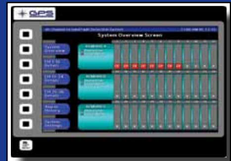
System Overview Screen
